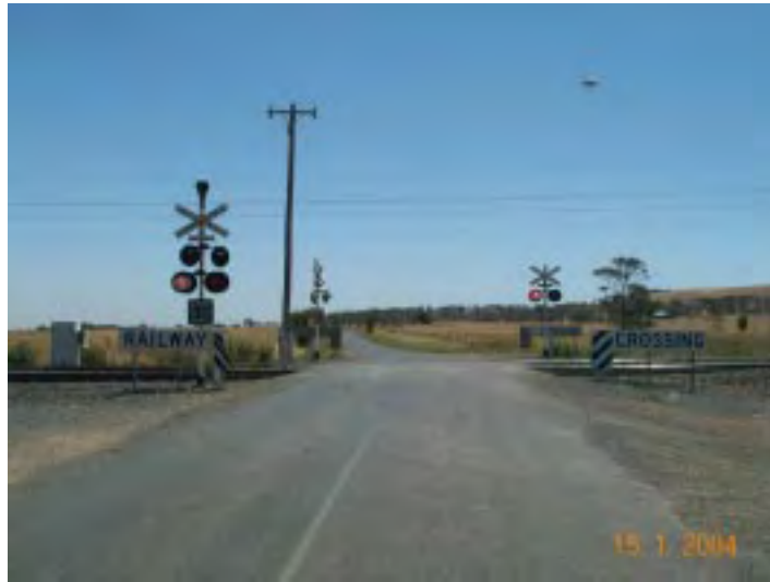
Flashing at the crossing
